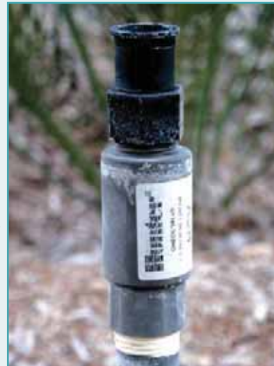
3. An in-line check valve can be used with the lowest nozzles on a slope to help prevent “low head drainage.”
