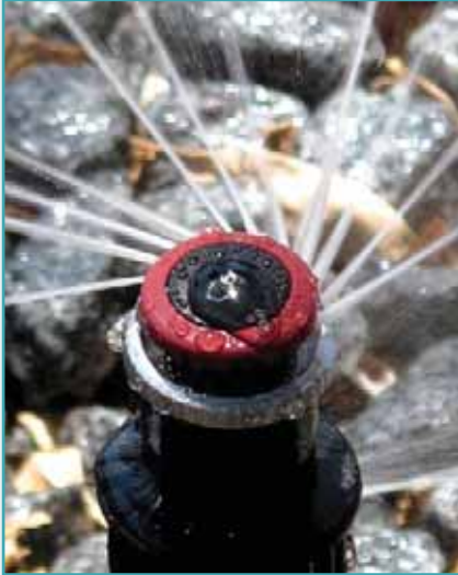
4. The small stream rotor nozzle is a new technology that can be easily retrofitted into most irrigation systems. They are more efficient and can result in some water conservation.
