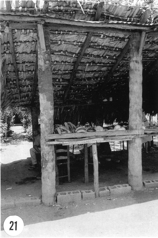
21. Posts cut from trunks of coconut palms being used as roof supports for roadside vegetable stall; leaves of "cana" used to provide roofing, 18 km north of Jarabacoa. (July 1, 1994). 22. Street vendor ("ambulante") selling hats made of leaves of obtained from the coconut palm ( Cocos nucifera ). (Samaná, Feb. 22, 1993).
