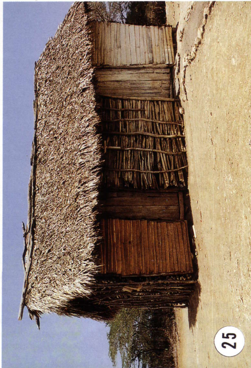
23. "Yagua" from the royal palm used as roofing for rustic pole frame structure, La Cantera, 3.2 km west of Río San Juan. (June 20, 1991). 24. House constructed with wall of "yagua" obtained from the royal palm and roof of leaves of "cana," 8 km south of Dajabón. (June 30, 1994). 25. House with thatched roof of leaves of "cana" obtained from the sabal palm. Front wall constructed of "cayuco," (a cactus) in center, and "tejamanil" (on right), 12 km east of Monte Cristi. (Sept. 23, 1992). 26. House roofed with leaf sheaths of "yagua" secured with poles tied to roof frame with "ripió;" house is sided with "tabla de palma," Yanu, 29 km northeast of Higüey. (June 25, 1989).
