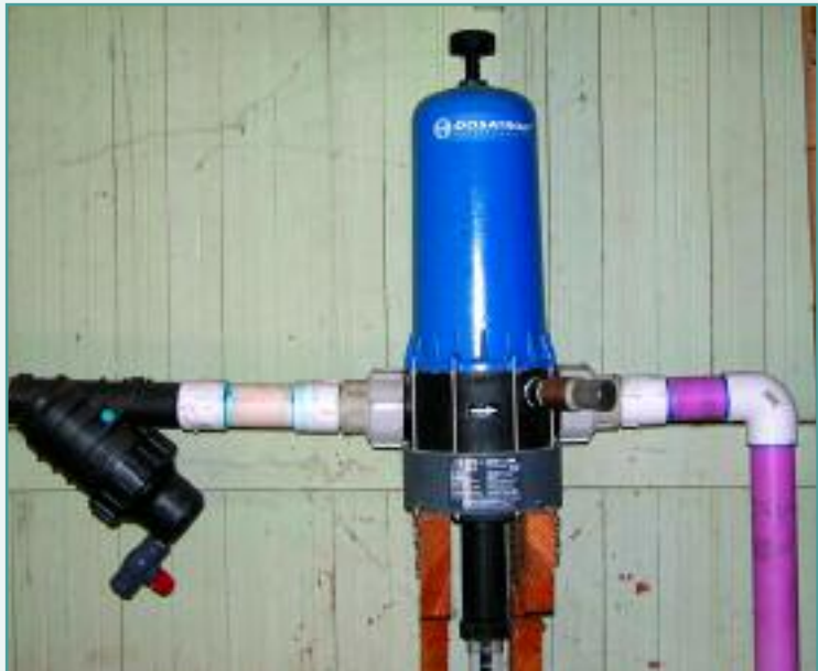
2. A 100 GPM Dosatron proportional fertilizer injector in use in the author's garden.
