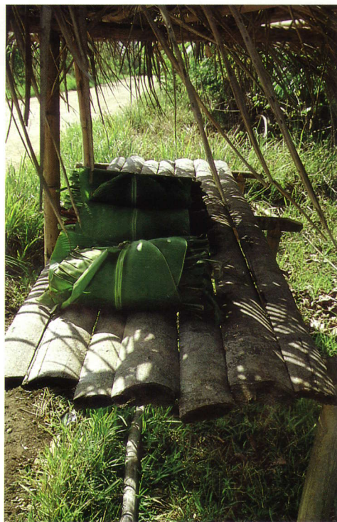
10. Upper. Roof corners are held in position with hollowed-out trunks of Veitchia macdanielsii , Olpoi village, west Espiritu Santo. 11. Lower left. Detail of house wall constructed of split trunks of Veitchia macdanielsii ; the black sclerotic fibers within the cortex of the trunk make an attractive pattern (Lakatoro, Malakula). 12. Lower right. Roadside food stall bench constructed of split trunks of Veitchia macdanielsii (Wormet, Malakula).
