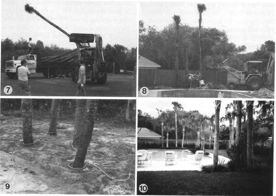
7. Unloading with a backhoe/front-end loader. 8. Setting the palms in place. 9. A simple temporary irrigation system. 10. The same landscape one year later.
