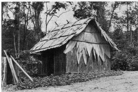
99. Leaves of Johannesteijsmannia are used for thatch and siding on a forest reserve building
