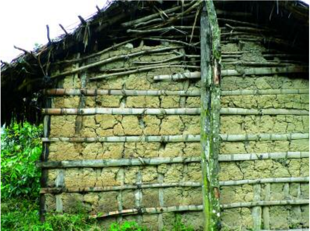
4 (top). Young plantation of Ceroxylon echinulatum for domestic use in an agroforestry plot, established from the seeds of the mature individuals visible in the background. 5 (bottom). Farm house showing the use of material from the outer part of the trunk of Ceroxylon echinulatum .
