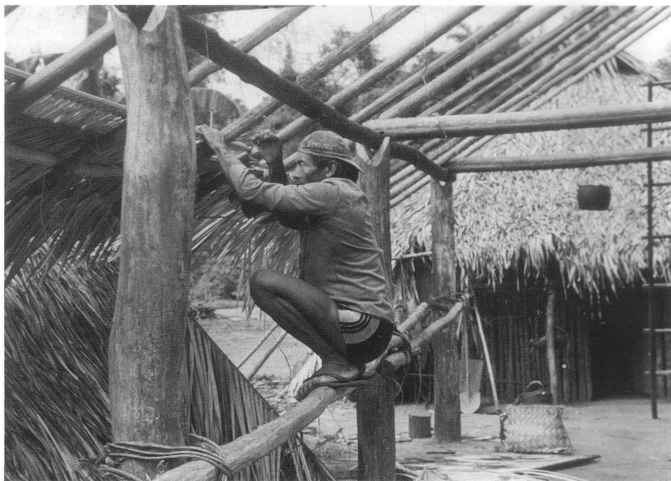
5. Asurini man thatching roof with leaves of babassu palm ( Orbignya phalerata ).
