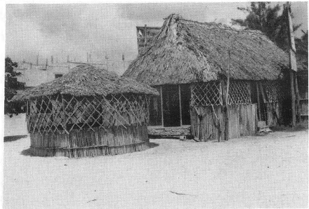
11. Rustic houses built with trunks of C. readii thatched with leaves of Sabal yapa .
