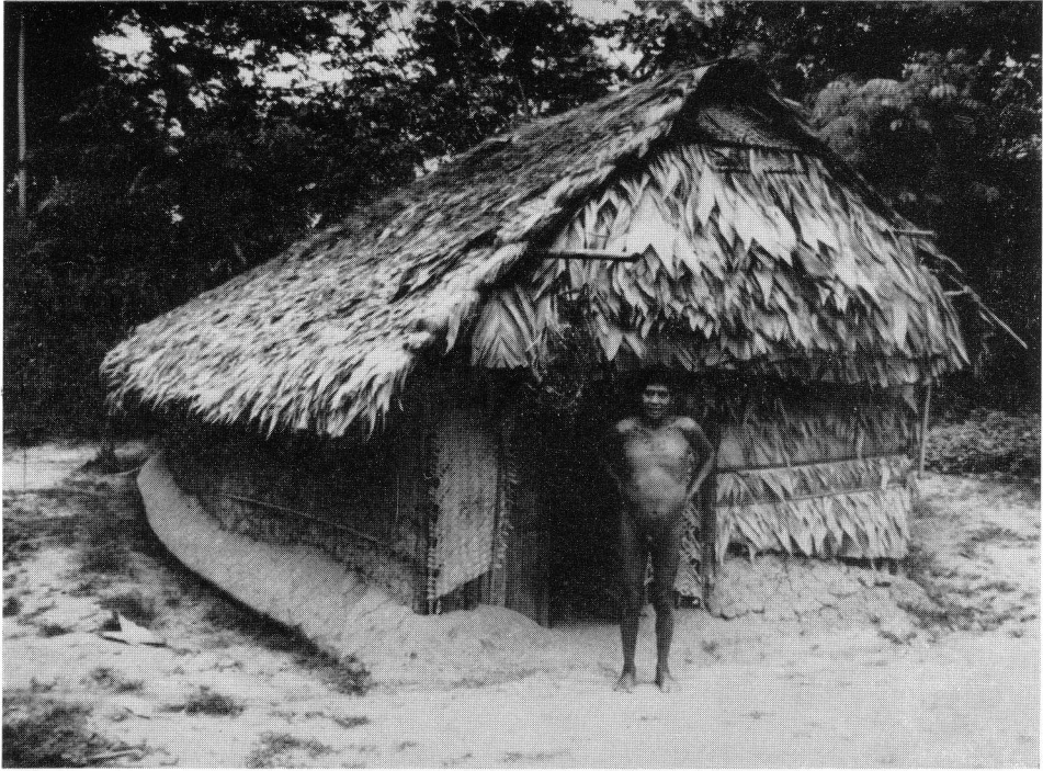
3. Dwelling with roof thatching made from leaves of bahanaki-siki ( Geonoma baculifera ); weaving adjacent to door made from leaves of okolaxi-siki ( Maximiliana martiana [ M. regia ]).
