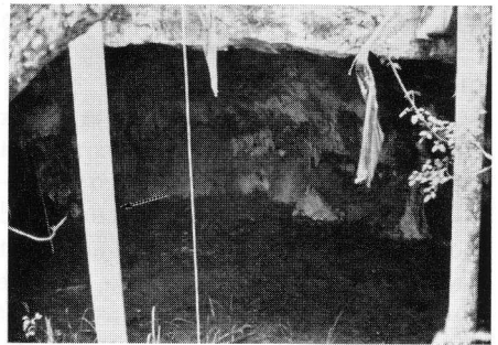
3. Interior of sinkhole showing organic soil and standing water. Arrow indicates royal palm trunk. To the right of the trunk is an aerial root of Ficus .
